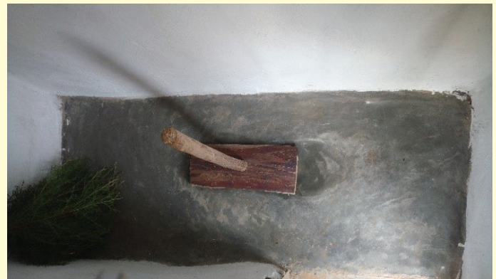
Interior of Agnes' Latrine
